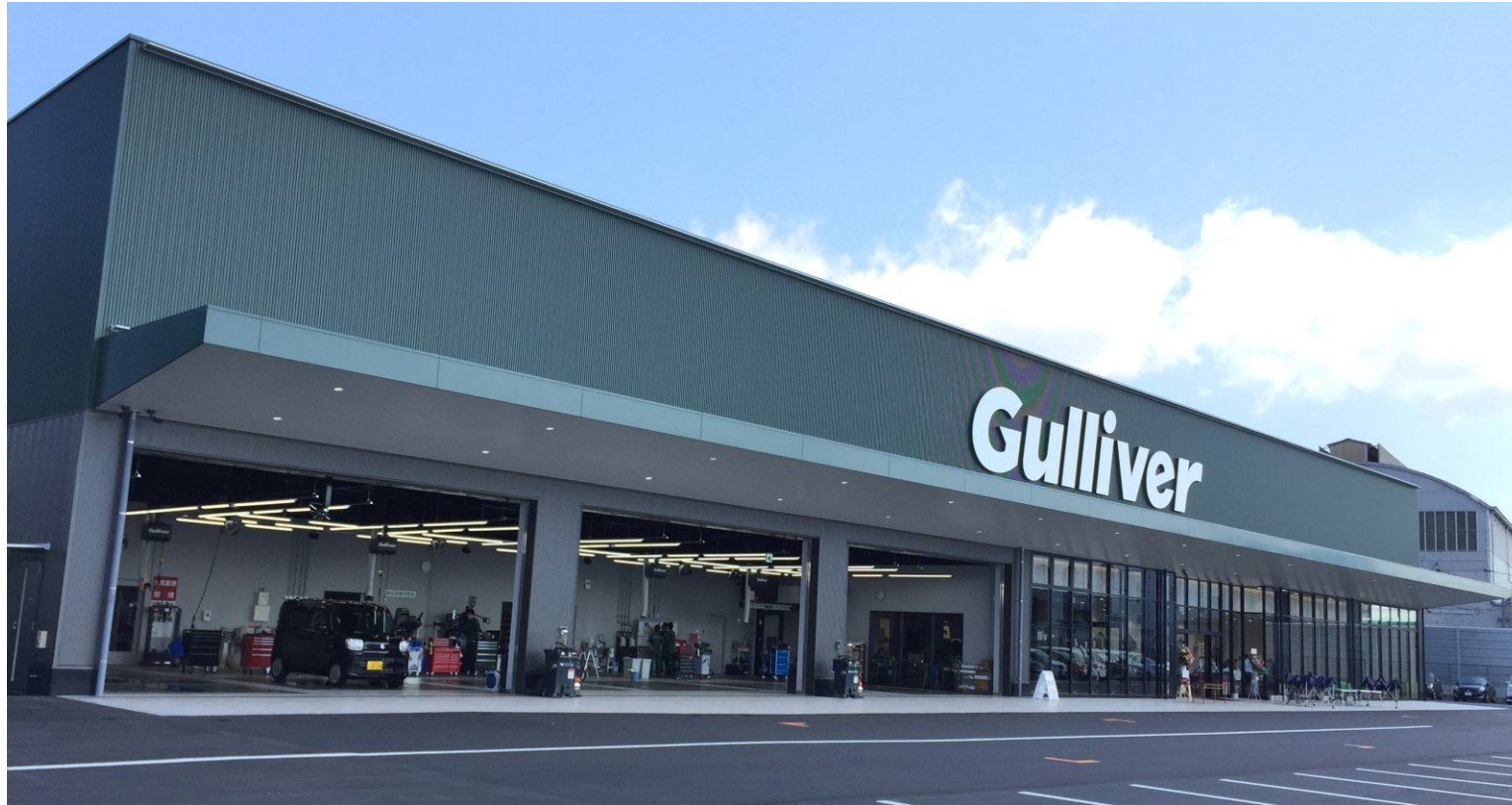
Kusatsuminami car maintenance shop (Opened in June 2022)
