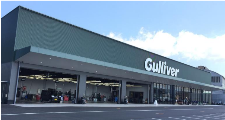
Kusatsuminami car maintenance shop (Opened in June 2022) Kusatsu-shi, Shiga Prefecture
