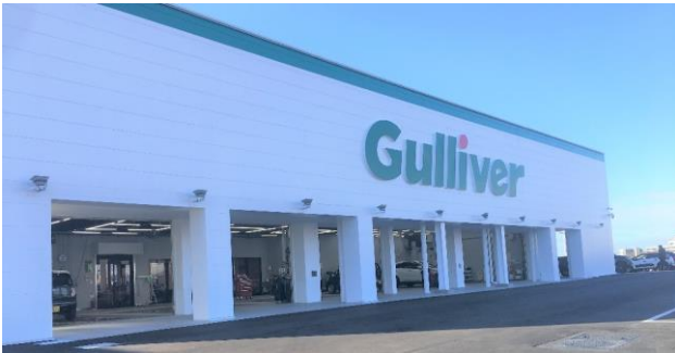
Himeji car maintenance shop (December 2021 Opened) Himeji, Hyogo
